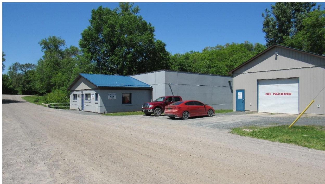
Figure 7 - Marmora Water Treatment Plant
