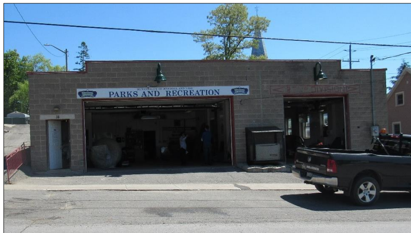
Figure 14 - Marmora Parks and Recreation Garage
