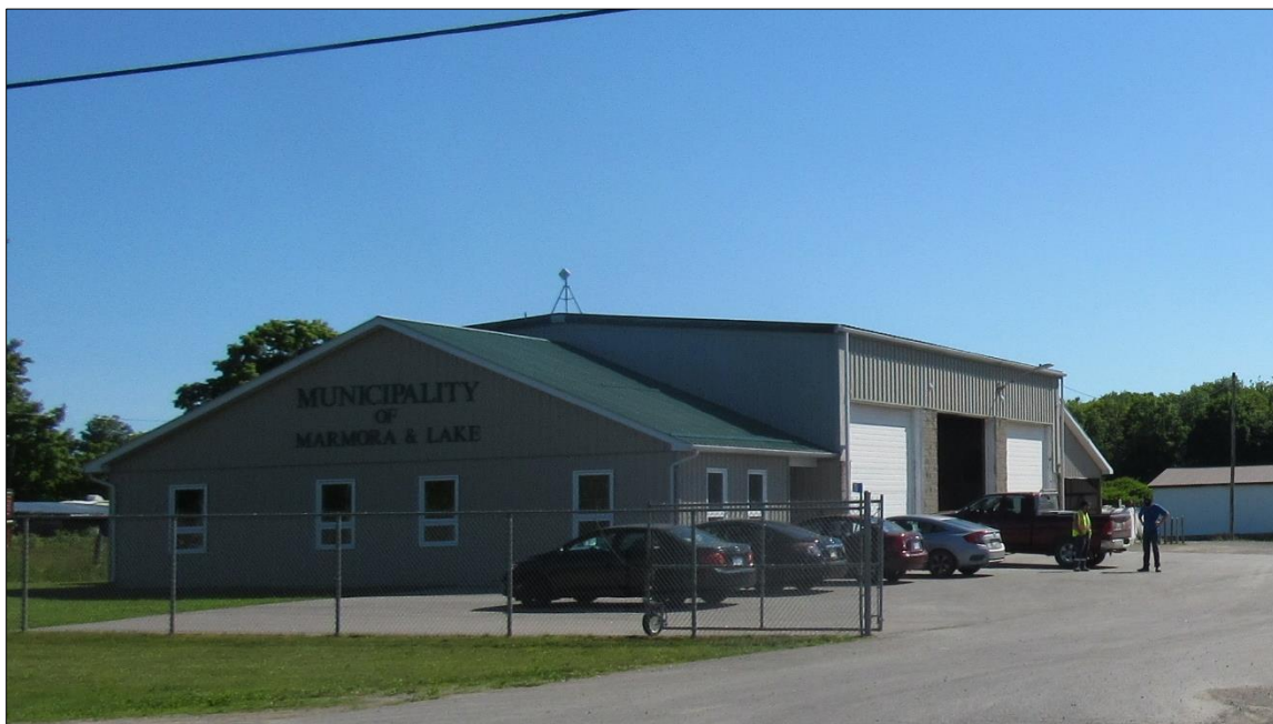
Figure 22 - Marmora Public Works Garage
