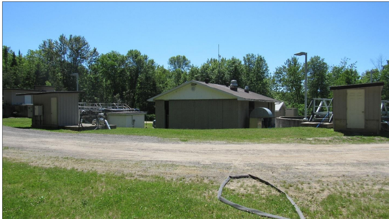
Figure 16 - Marmora Waste Water Treatment Plant
