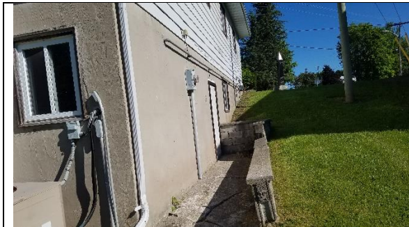
Figure 42 - Emergency exit of east face
