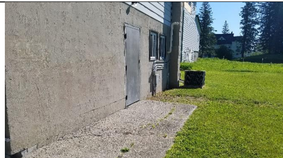
Figure 43 - Rear exit door
