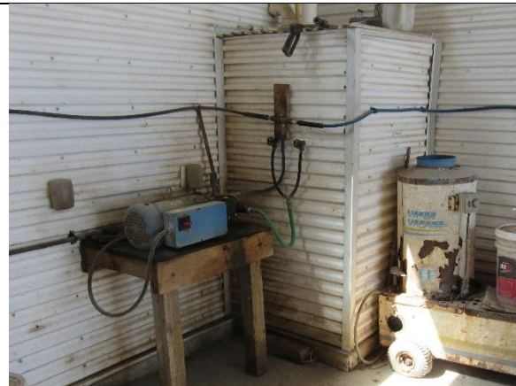
Figure 24 - Concealed HWT in wash bay
